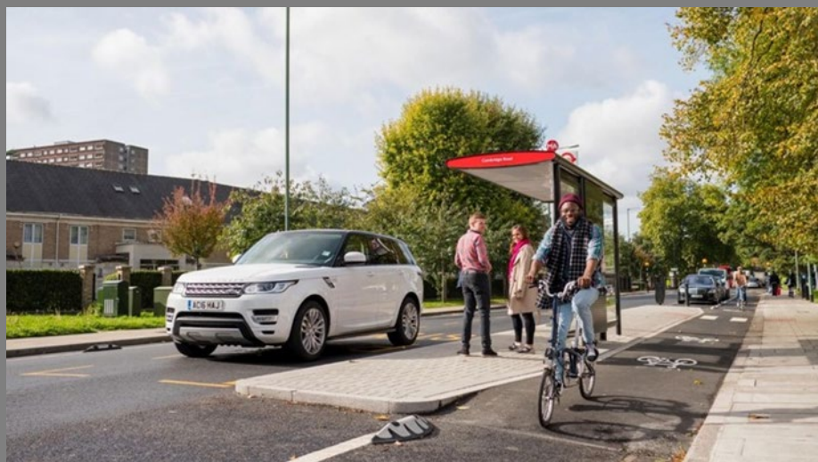
Figure A1-7: Example of protected bike lane.
