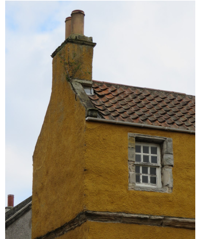
Rendered chimney and pantile roof
