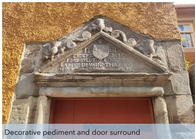
Historic door and masonry surround
