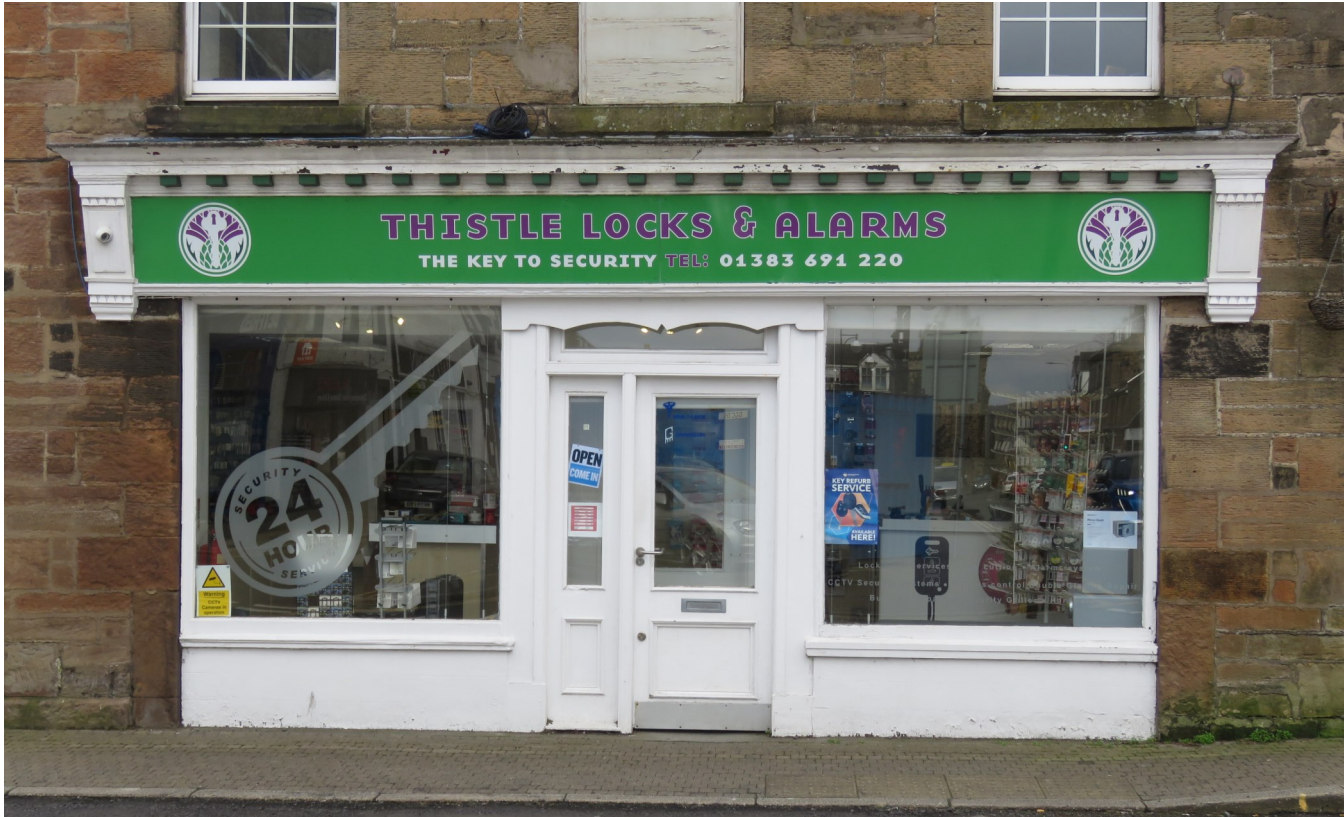
Surviving Inverkeithing shopfront with fascia, dentilled cornice, and console brackets
