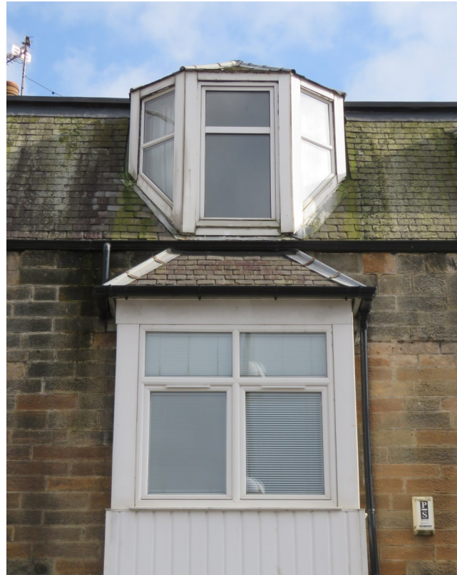
UPVC dormer and oriel window – would not meet current standards of good conservation practice
