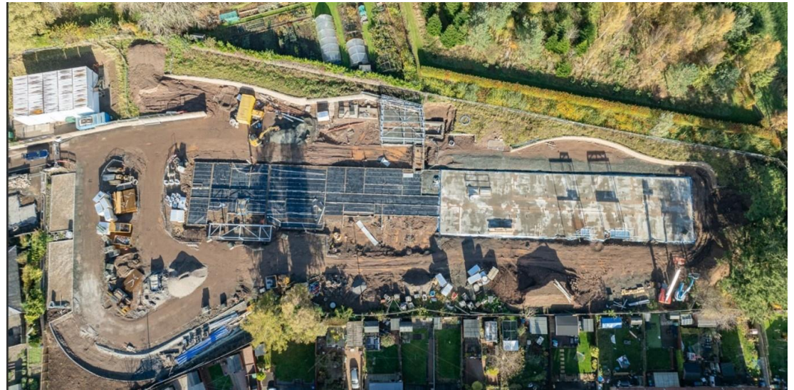
Work underway at Cupar Care Village
