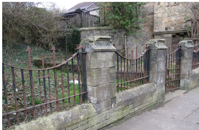
Boundary and railings to former Primary School
