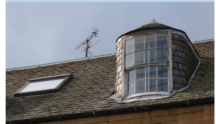
Traditional dormer and rooflight (not flush – would not meet current standards of good conservation practice)
