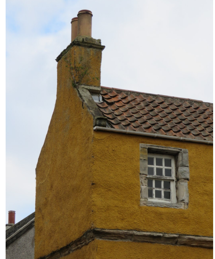
Rendered chimney and pantile roof
