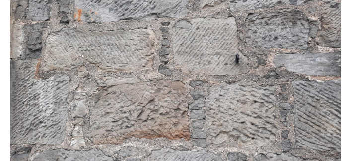
Ladder pinning at the Town House
