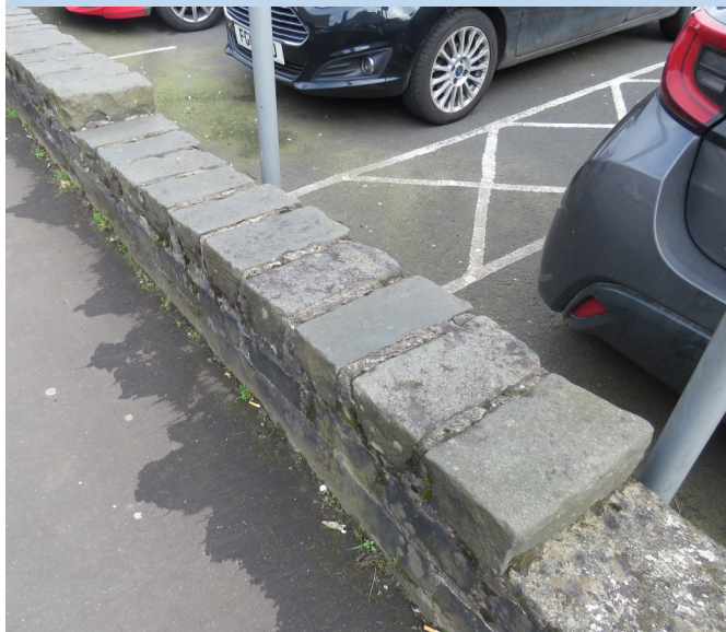
Wall made of stone setts
