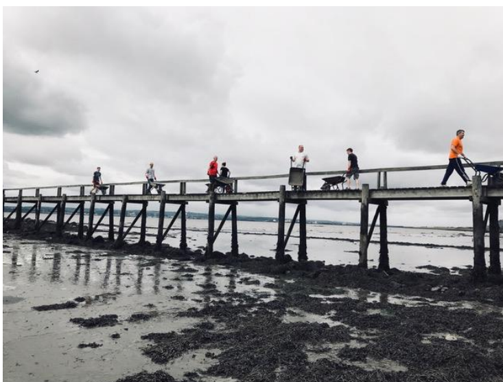
Figure 2 - An image of the work being undertaken to restore Culross Pier
