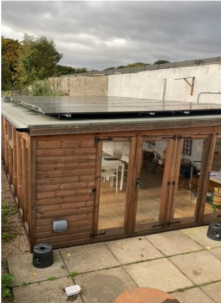
Figure 7 - The Grow West Fife sustainable kitchen with solar panels
