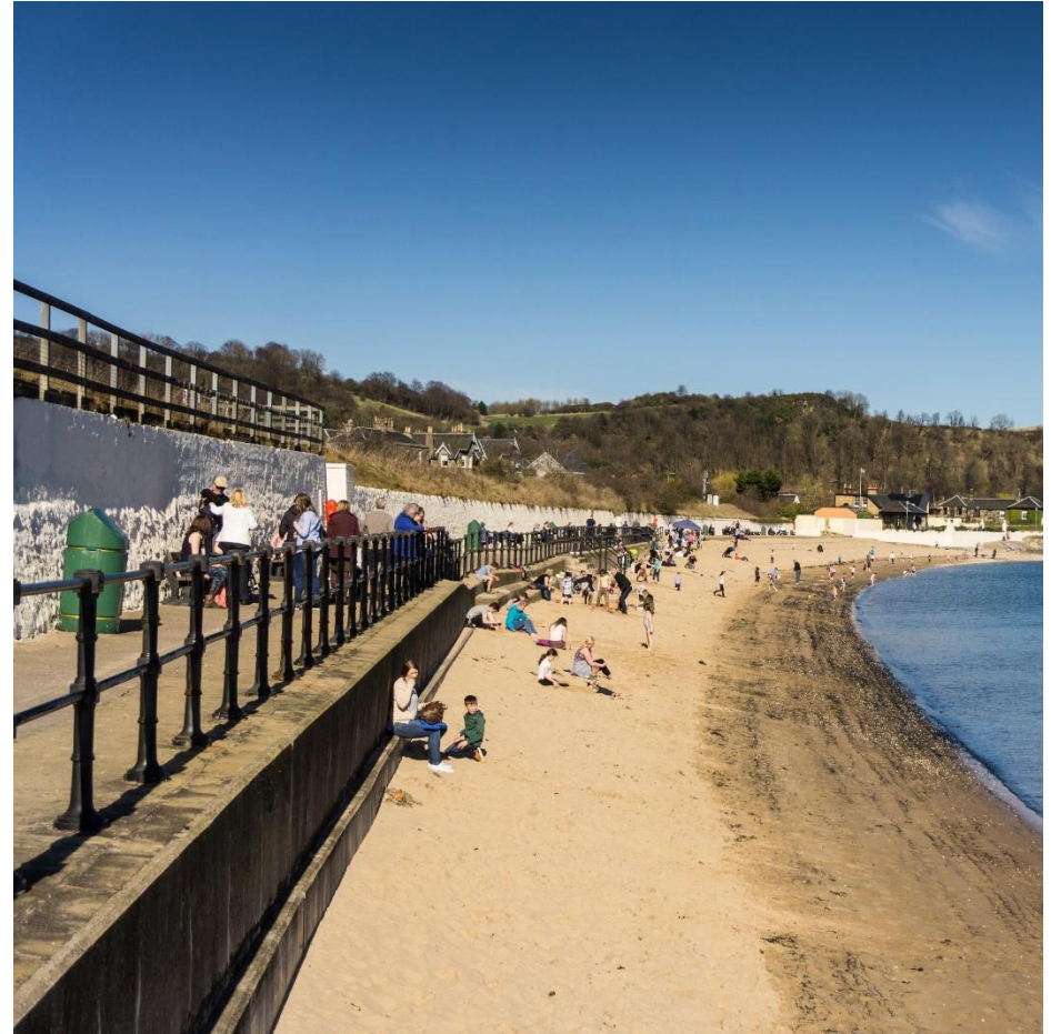
Burntisland beach showing how the railway embankment cuts off the town from the coast
