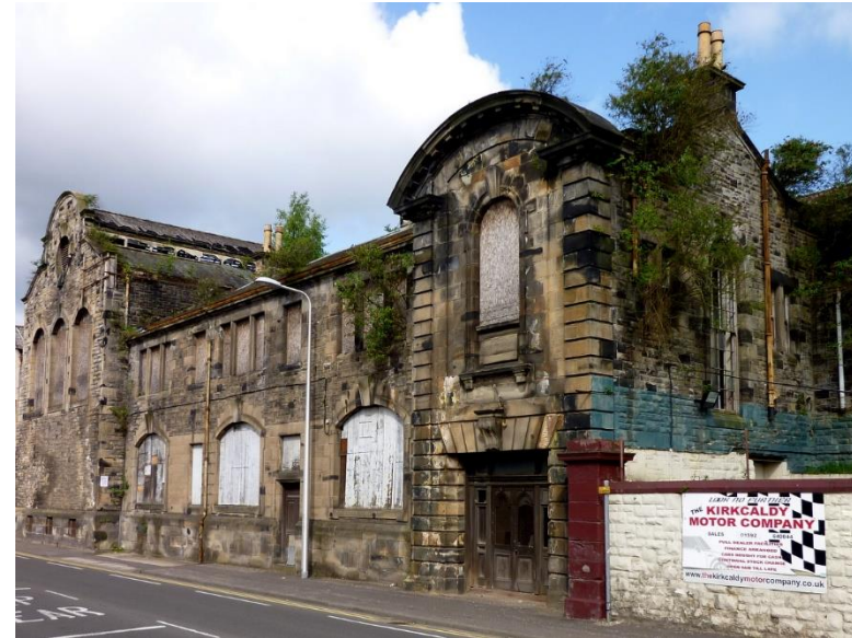
B Listed Victoria Road Power Station, Kirkcaldy – now demolished
