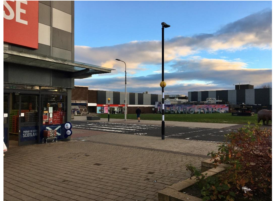
Glenrothes Town Centre - looking across North Street to the Kingdom Centre and new temporary locality of greenspace created on the site of a demolished office building
