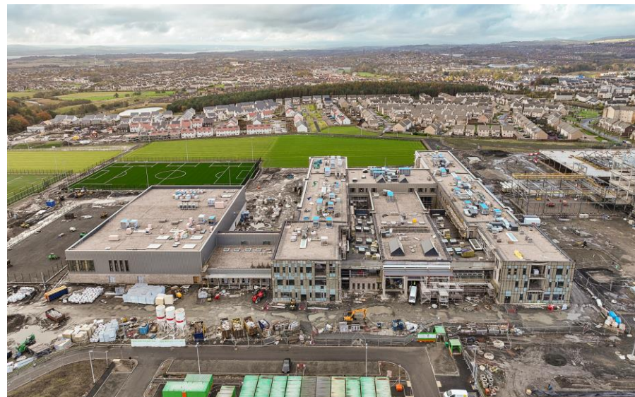
An aerial view of Dunfermline Learning Campus under construction
