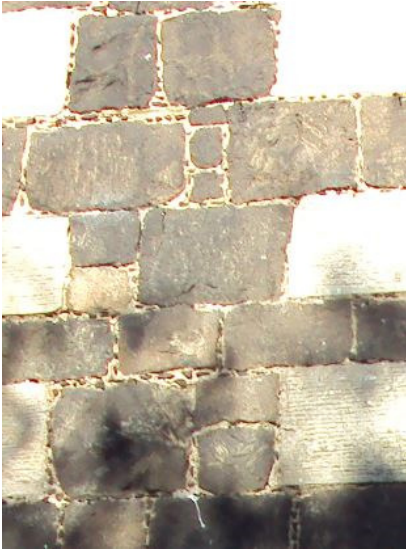
Coursed square whin rubble laid in Aberdeen bond style with cherry cocking pinnings and sandstone freestone margins (Manse).
