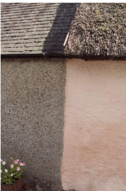
Contrasting modern cement render with softer more traditional finish.
