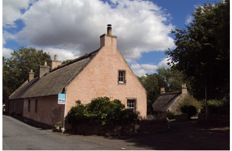
Traditional lime wash
