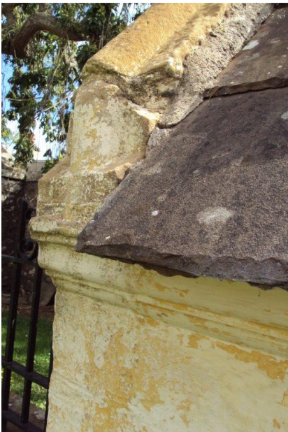
Traditional lime wash
