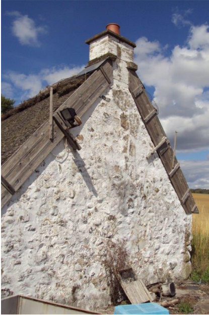
Traditional lime wash
