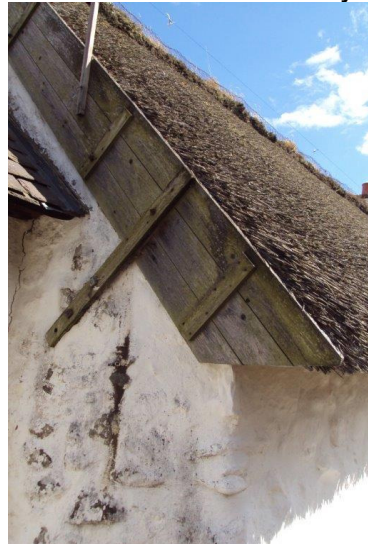
Gable board (above left) and turf ridge (above right) thatch details.
