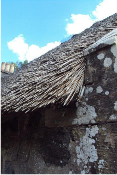
Eaves and raised gable wall head detail.
