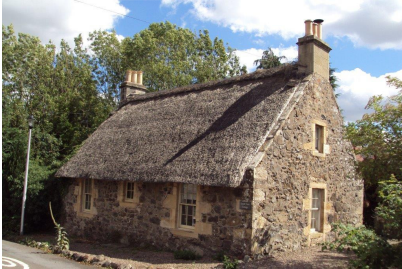
Southview above has had the felt tiled roof replaced with thatch.
