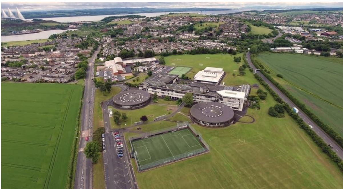
Figure 7 Inverkeithing High School
